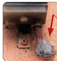
Corrugated pipe entry protection
